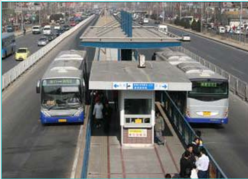
Beijing – Southern Axis BRT line 1
