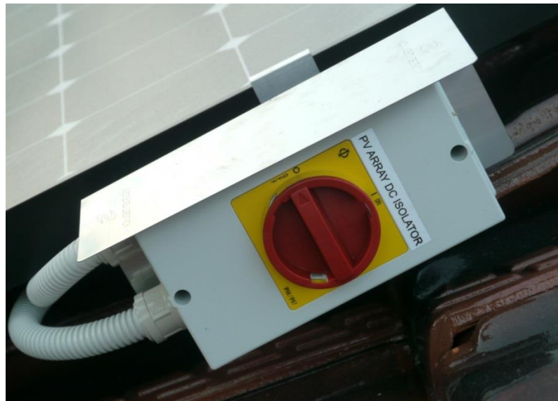
Figure A5: Shroud installed over rooftop isolator at the array
