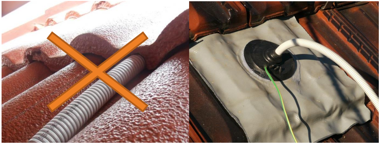
Figure A8.2. Left: wiring system penetration incorrectly installed between tiles. Right: wiring system penetration correctly installed with vertical penetration using a collar flashing.
