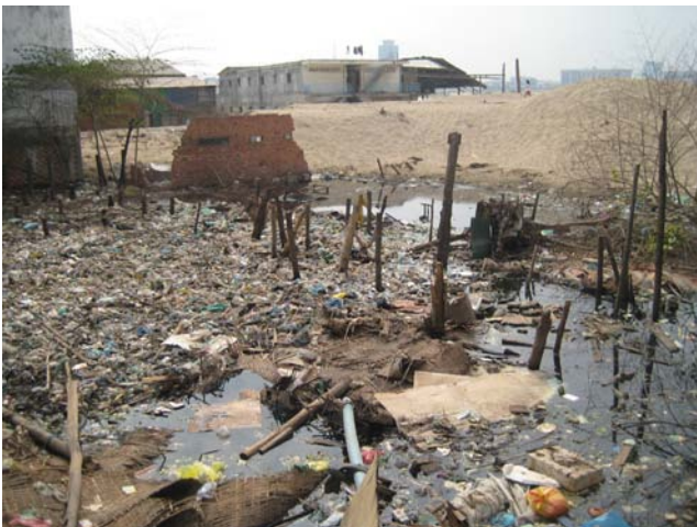
Above and right: Phnom Penh houses demolished in forced evictions
