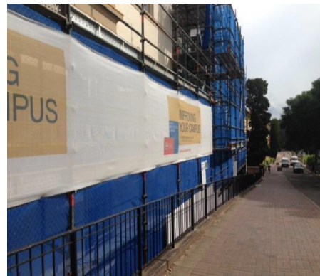
Image 6 - Example of Shade Cloth Sign on Scaffold
