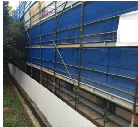
Image 4 - Scaffold with Hoarding and Cloth
