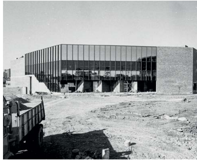
The Seymour Centre under construction, 1974
