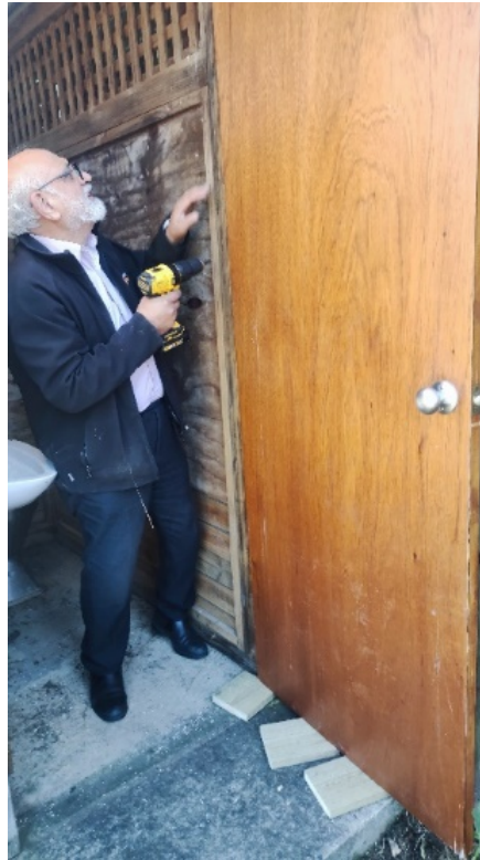
Iqbal installing new door to bathroom
