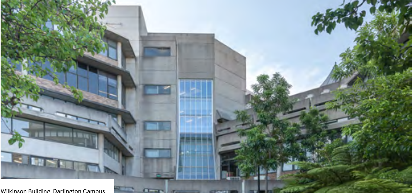
Wilkinson Building, Darlington Campus
