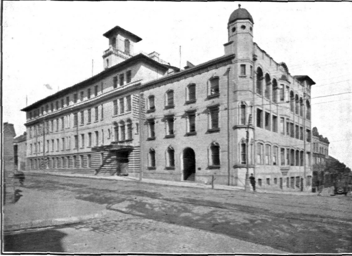
CROWN STREET WOMEN'S HOSPITAL.
