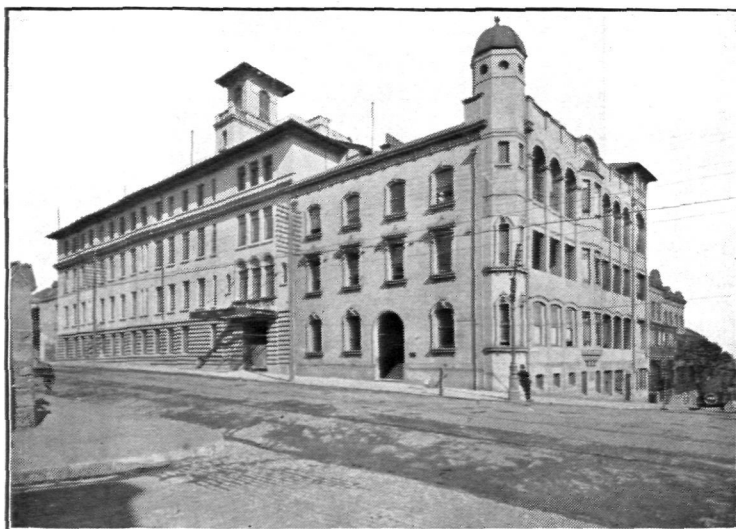
CROWN STREET WOMEN'S HOSPITAL.
