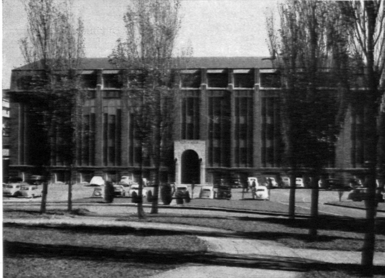
The New Medical School as it is at present.
