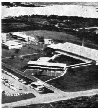
The Abbott plant on Captain Cook Drive, Kurnell.
